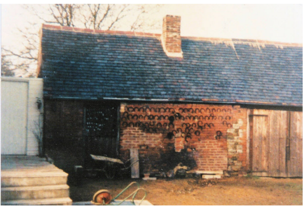
The forge in Gilks Lane, before demolition
